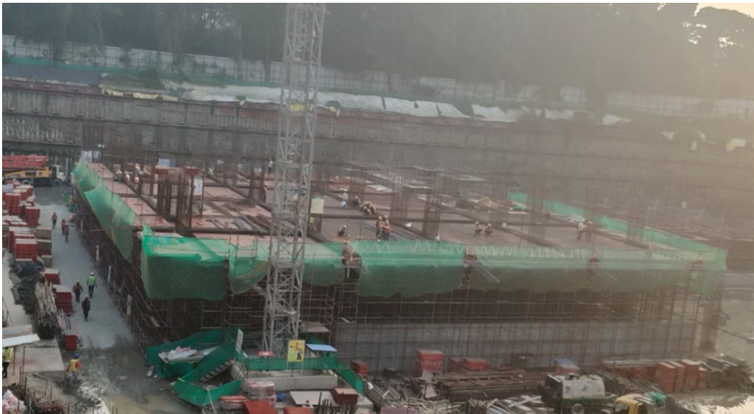
Construction status Photographs
