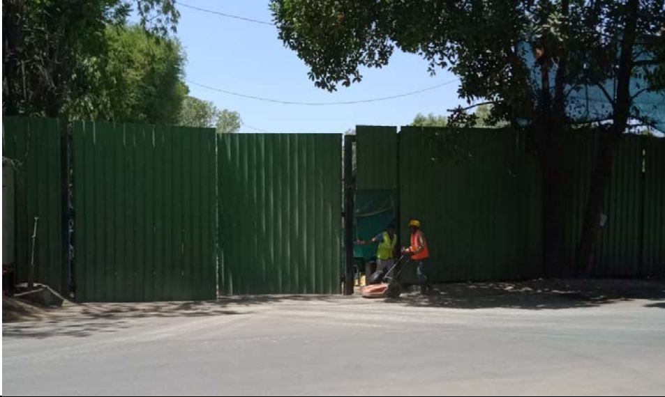
Entry- Exit gate
